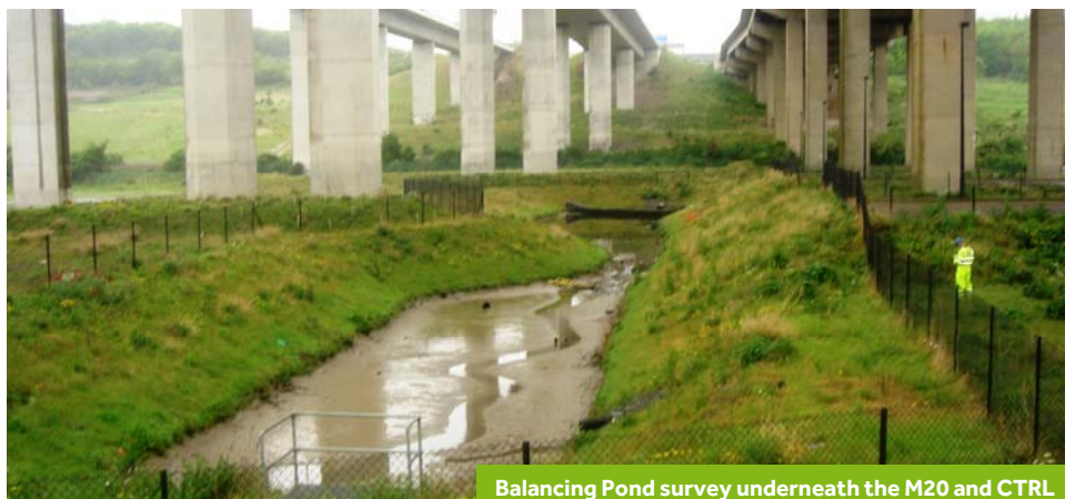
Balancing Pond survey underneath the M20 and CTRL
