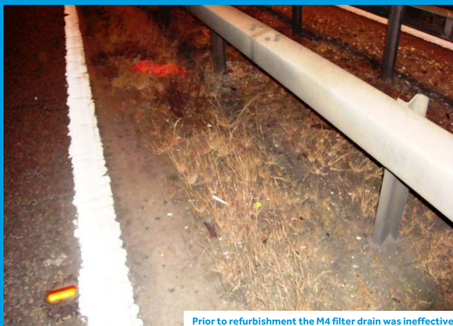
The M4's newly optimised drainage system
